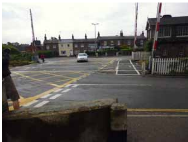
Looking south across the level crossing
